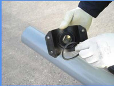
3. Couple the bottom part of the saddle with the upper one. Insert the bolts from the bottom, screw
